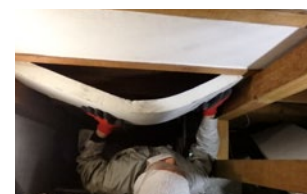
Achilles Juten R being installed
