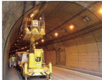
We offer the Tn-p Construction Method, effective in maintenance and repair of older tunnels with age-related degradation, nationwide in Japan. This tunnel maintenance and repair technology (backfill injection) prevents tunnel collapse and damage from events such as earthquakes by injection filling Achilles Aeron-R (urethane foam) into voids that form behind the lining of older tunnels.
