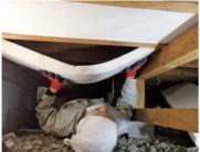
'3 With thermal conductivity of 0.018 W/(m K), panel thickness has been reduced to 29.5 mm to enable insulation during remodeling with minimal reduction in the size of the interior space.
