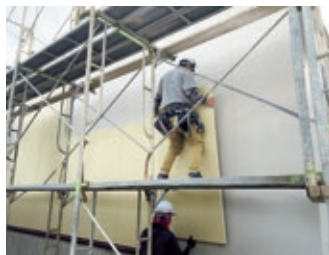
View of “QD Panel Steel Frame External Insulation System” being installed
