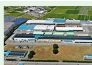
Shiga Factory No. 2, Achilles Corporation
