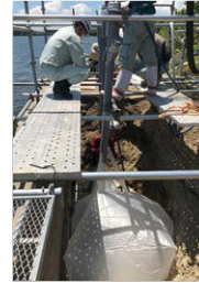
Infrastructural civil engineering method: "Juten-bag method"
