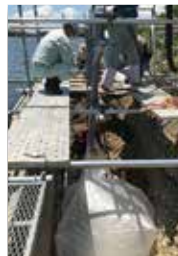
Infrastructure civil engineering method: "Juten-bag method"
